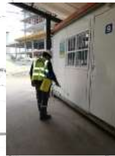
Personal hygiene with constant hand washing with soap and drinking water, provision of alcohol gel. Intensification of camp cleaning and disinfection frequencies
