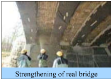
Strengthening of real bridge
