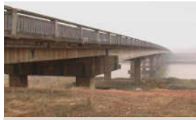
Shuiduhe bridge in Changsha
