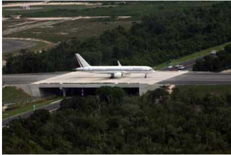
Road Works in the Cancun International Airport
